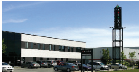
Montreal, Canada Manufacturing Center & R&D
